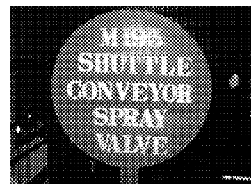
M195 Shuttle Conveyor Spray Line Signage
