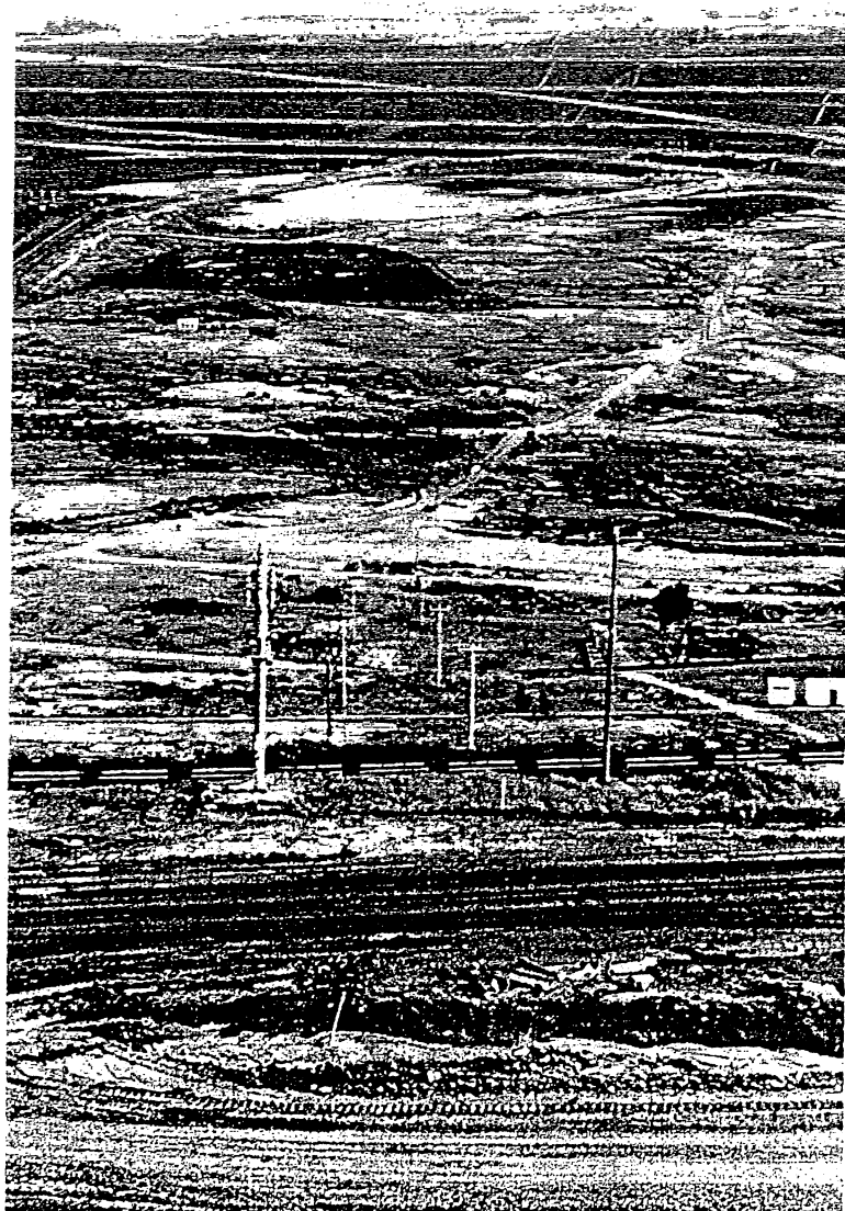
FIGURE 9: Looking north over "20 series" conveyor and along feeder lines 16 and 4 crossing the worked-out area, predominantly on timber poles.
