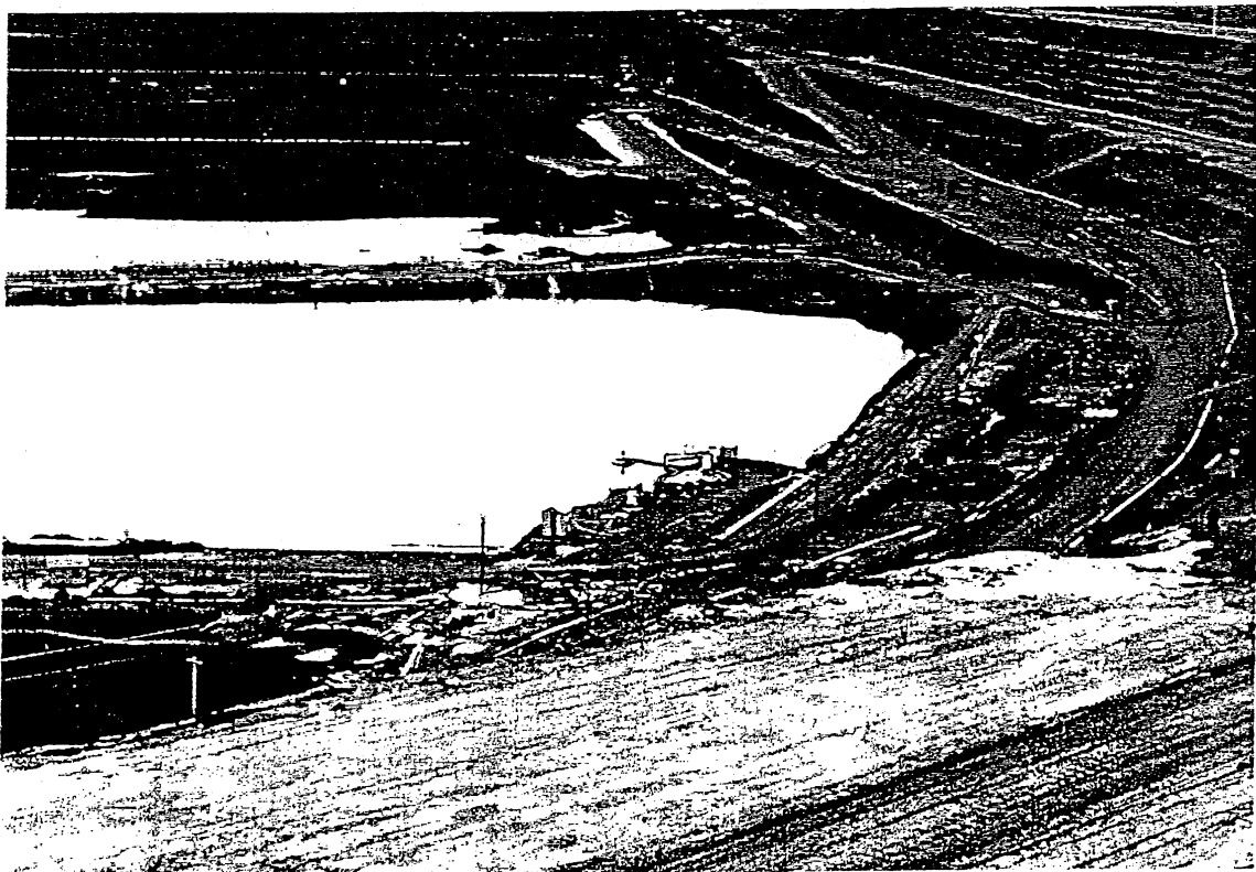
FIGURE 17: "H Section" located on grass level above the mine for valve control and mixing of clean and dirty water. Looking along the clean water line towards the mine, dirty water main on the right.
