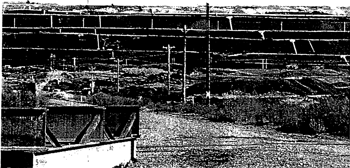
FIGURE 11: Feeders 15 and 16 crossing nearly through the middle of the worked-out area on timber poles, looking east.
