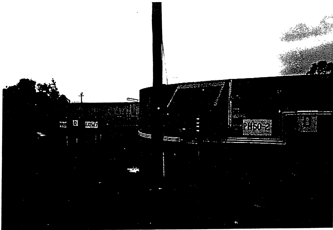
FIGURE 16: 100,000 gallon clean and dirty water tanks located near Hazelwood power station, for fire water storage and pressure control of the M.O.C. fire protection system.
