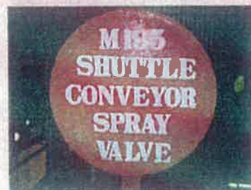
M192 & M195 Shuttle Conveyor Spray Line Signage
