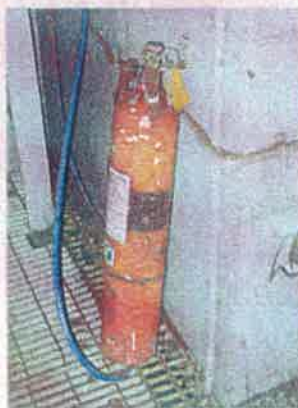
Control Room Walkway
