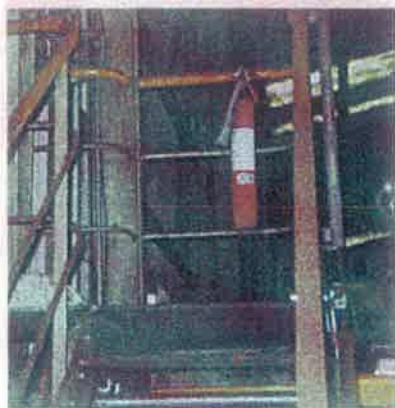
Lift Access Walkway
