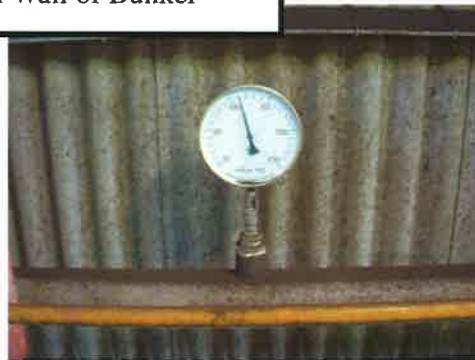
Pressure Gauge Located on Western Wall of Bunker
