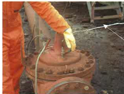
Water Release from Drain pipe Valve Turning ON
