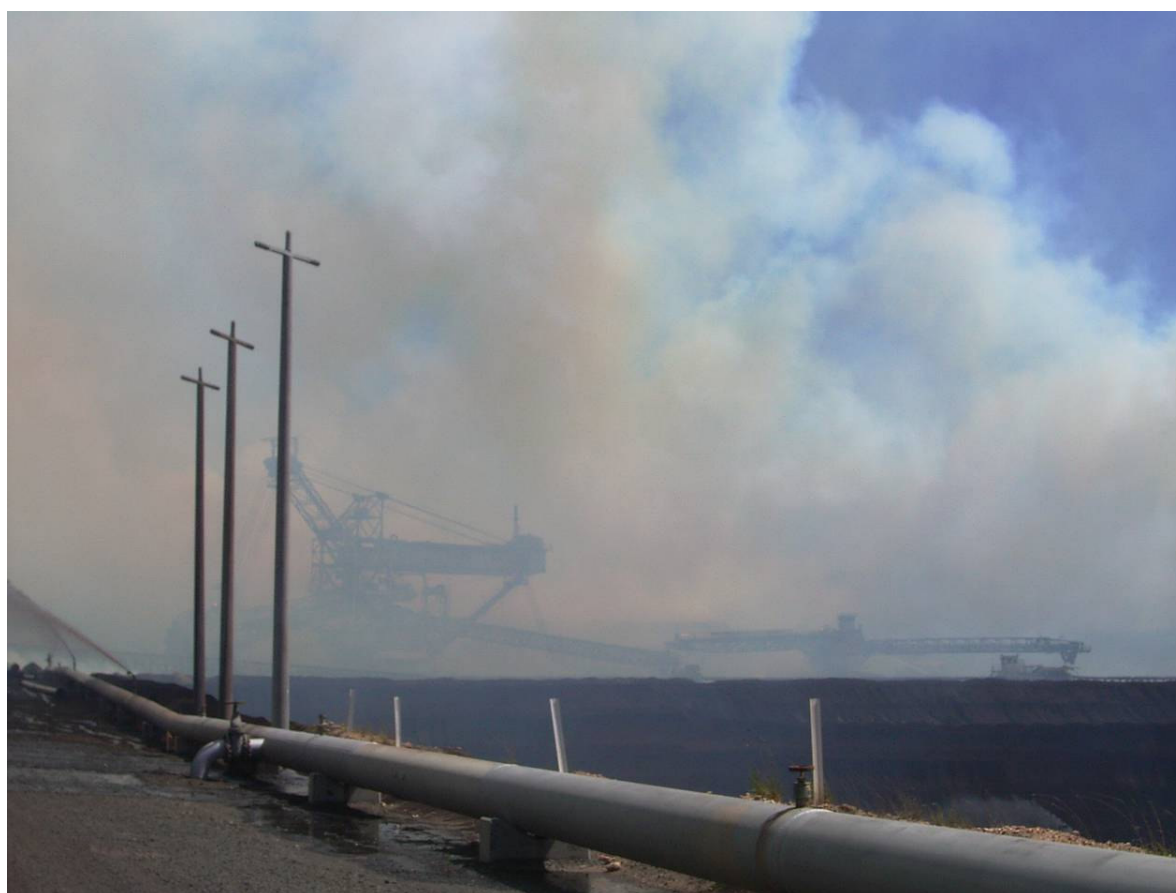
Dredger DR11, 12 October, 2006 – CFA Fire Investigation Team
