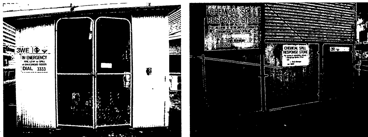
Figure 19 — Bunded chemical store (left) and chemical spill station (right)
