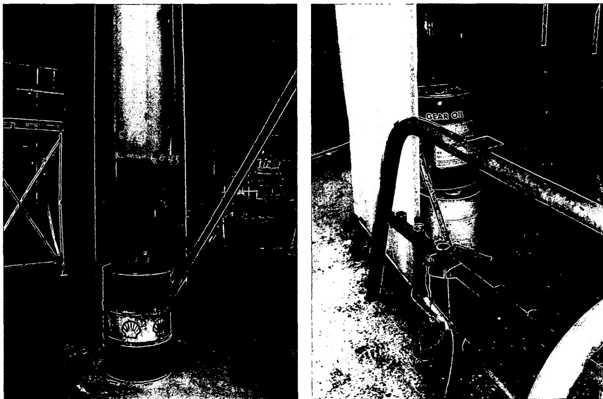
Figure 29 — A drum used to collect waste oil (left) and two small drums of new oil (right) under the boiler area
