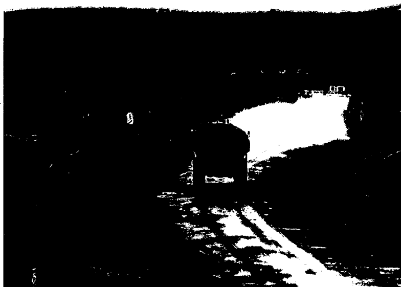
Figure 3 — Use of water truck to reduce dust. Note the lack of dust from the heavy vehicle travelling on the watered roadway
