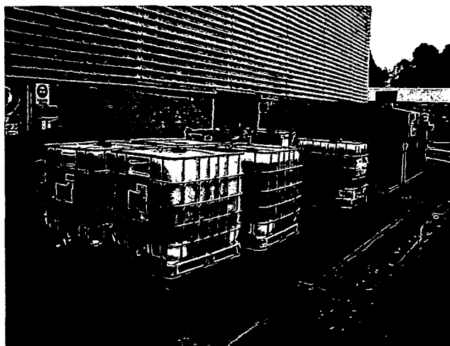
Figure 27 — Palecons of anti-scaling chemical stored along the roadway opposite bulk alum tanks
