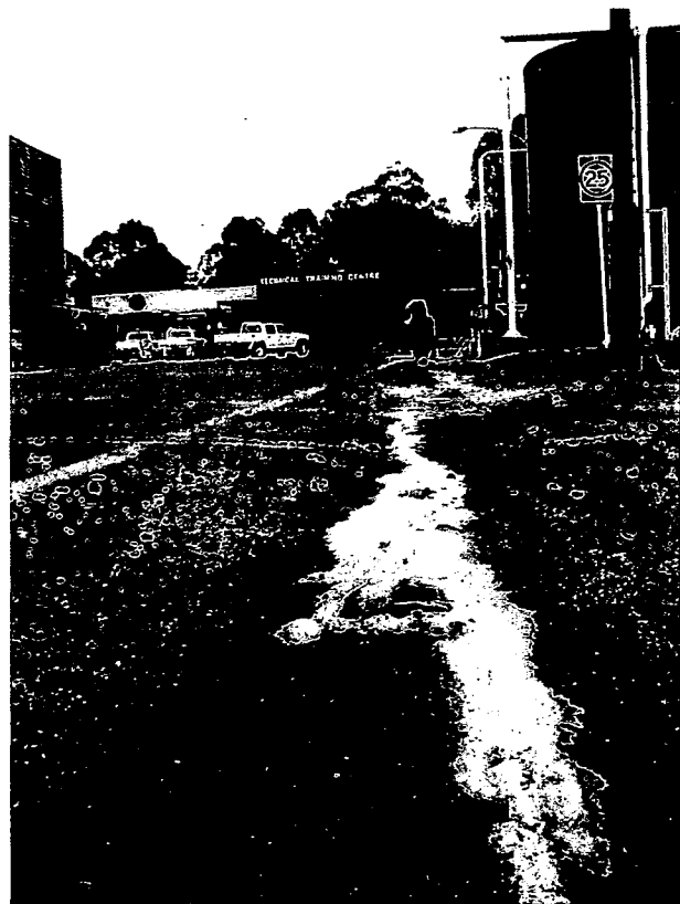
Figure 26 — Note spill of material on roadway following unloading (right). Unbounded alum and brine tanks (above)
