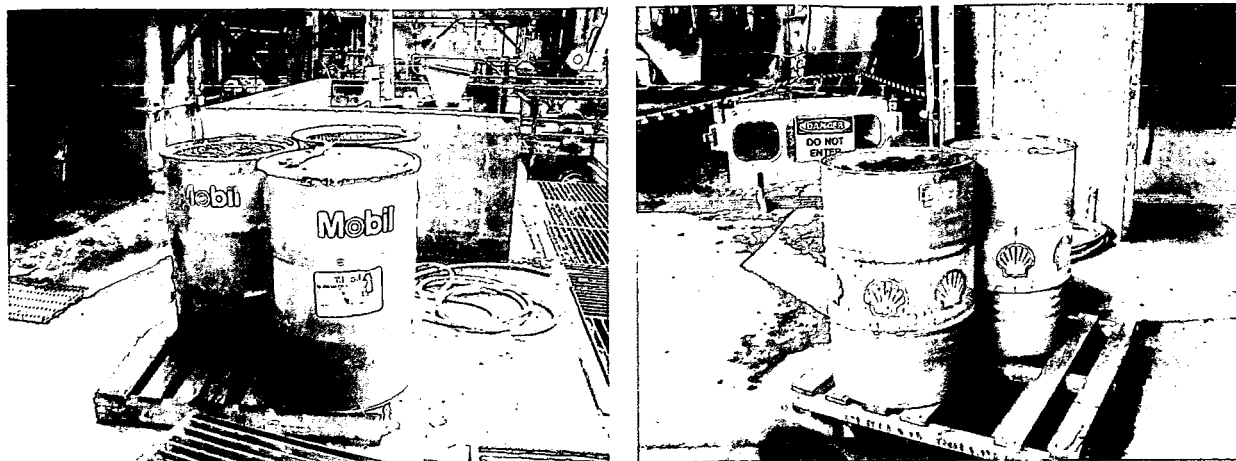
Figure 30 — Drums of waste oil (left) and a drum of waste oil - one drum is empty (right) under the boiler area
