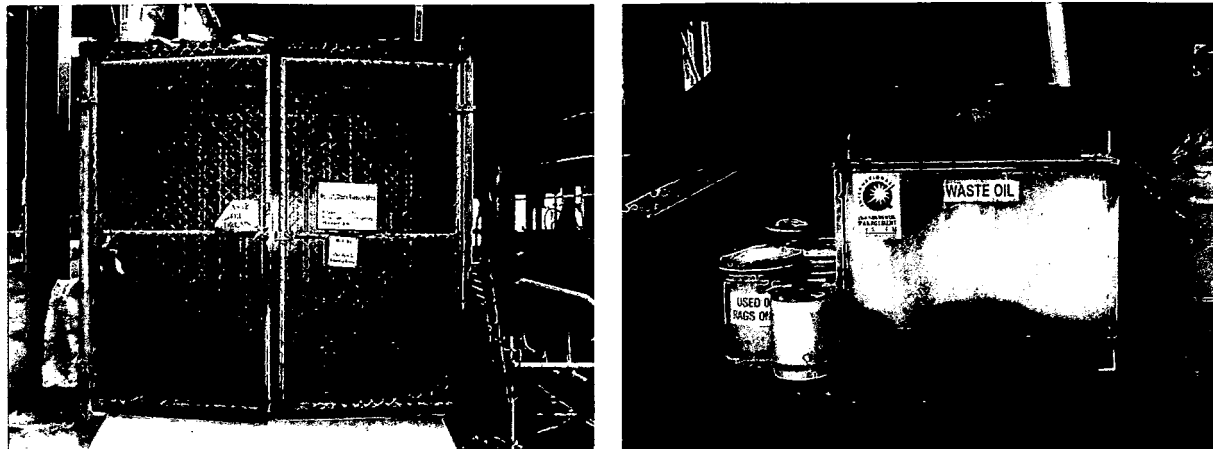
Figure 17 — Bunded "New Oil" enclosure (left) and waste oil and rags bund (right)
