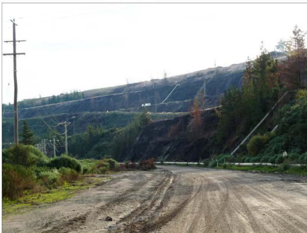
Figure 8: Vegetation on batters 16 May 2014
