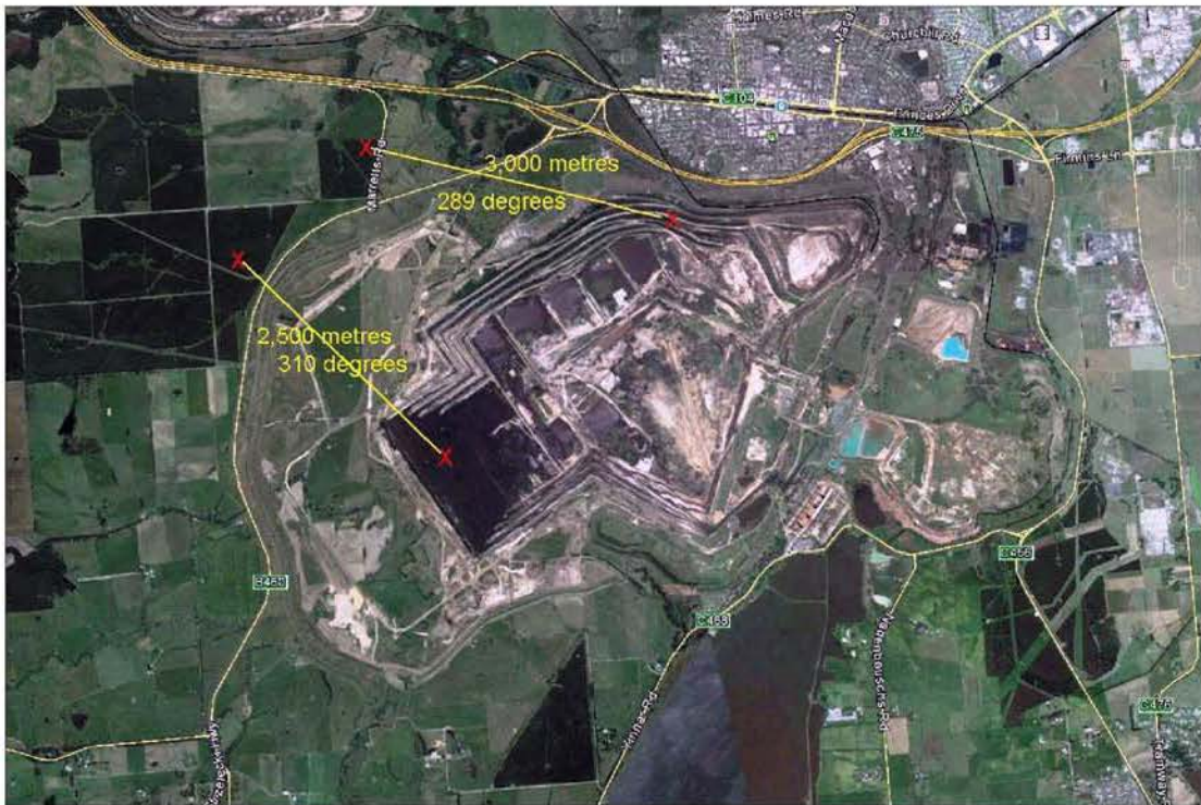
Figure 12- Distance of established eucalypt plantations from Hazelwood Mine (Google Image)
