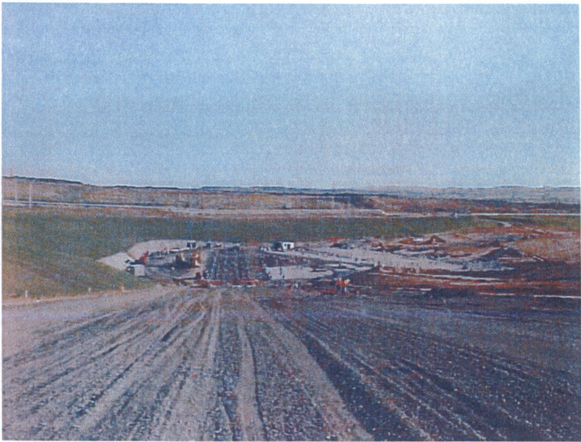
Part of Mine Permanent Void Batters (TP8 Area) 'Progressive Rehabilitation' work.
