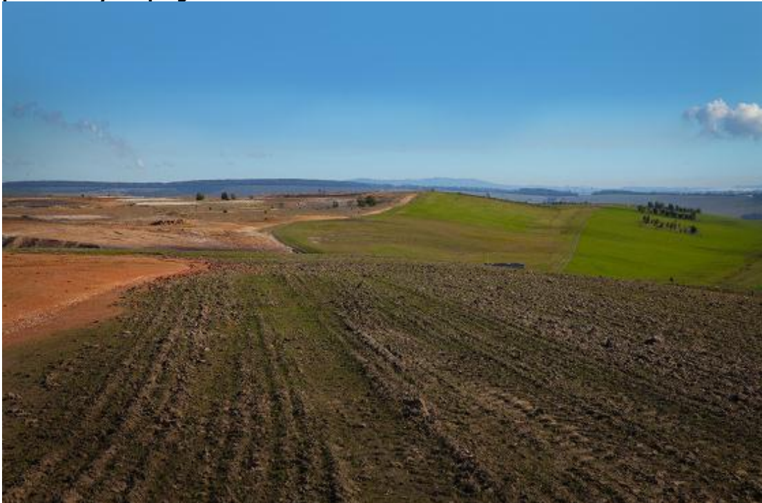
Plate 6 - Progressive rehabilitation landform – active mining face of the northern slopes contrast with final landform and land use; looking north.
