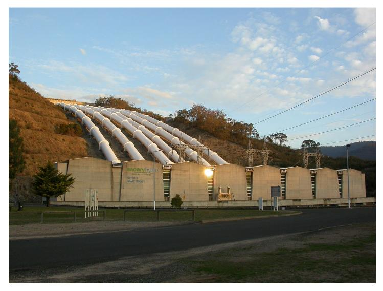
Tumut-3 Power station in the Snowy Mountains: Each penstock feeds a hydro-generator and the water is then collected in the Tumut reservoir below the turbines and pumped back up to the Talbingo Dam using off-peak electricity.
