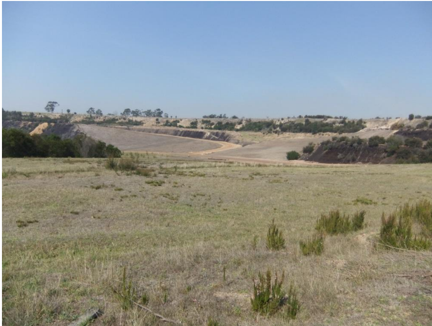
Figure 6: Topsoil Coverage (Feb 2015)
