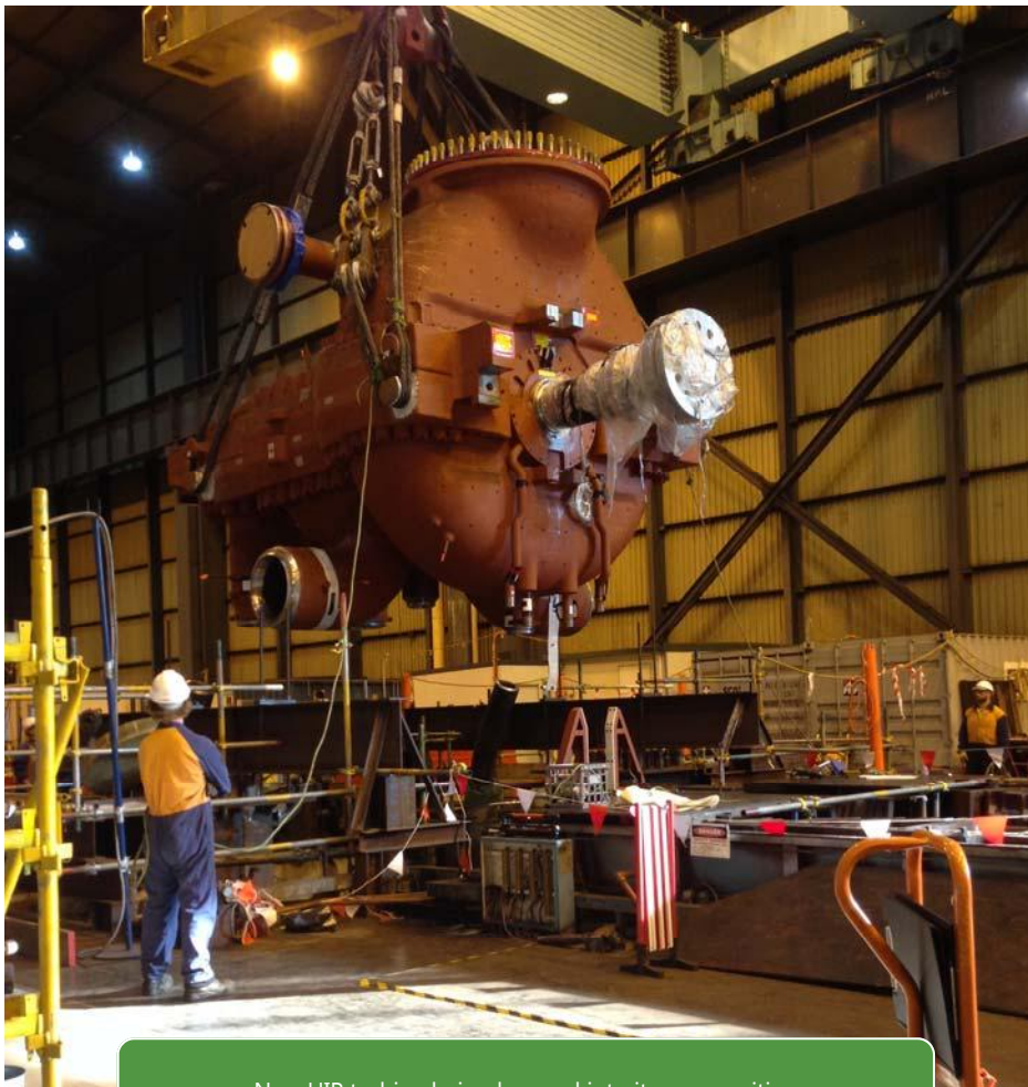
New HIP turbine being lowered into its new position
