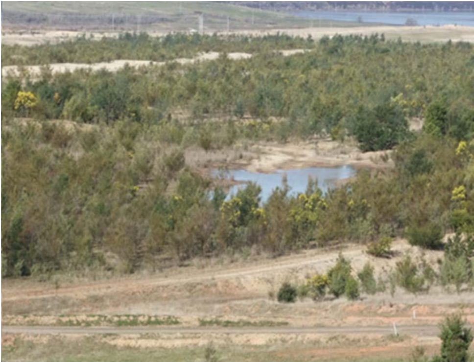
(a) Interim Stabilisation of Overburden Dump
