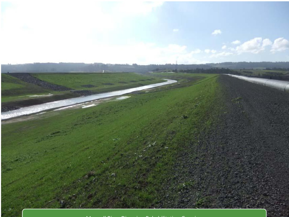
Morwell River Diversion Rehabilitation Grassing
