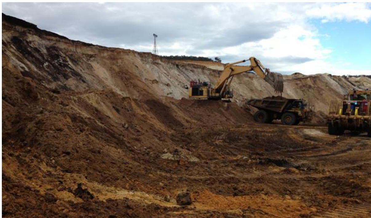
Figure 3-8 : Source of Capping Material
