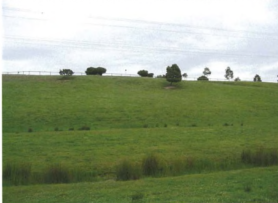
Plate 4 - Final rehabilitated landform - mine western batters –Viewing Mound
