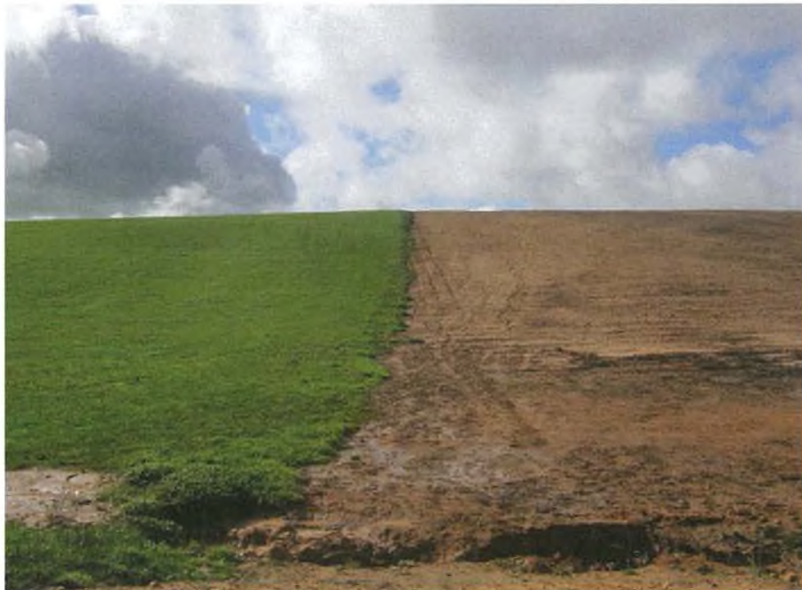
Plate 8 - Progressive rehabilitation landform – with topsoil and grassed and preliminary shaping.
