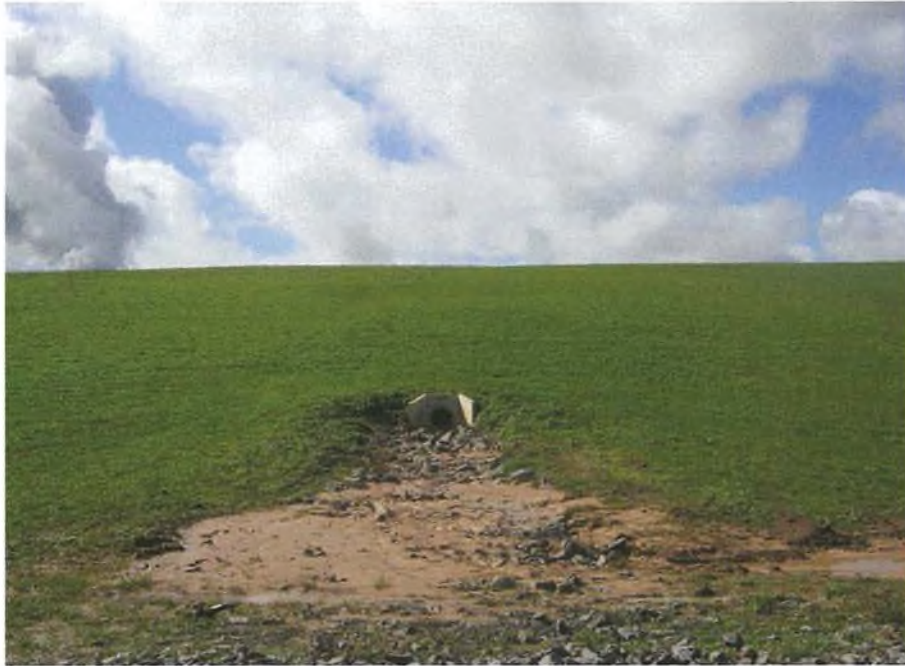
Plate 7 – Progressive rehabilitated landform – down slope drainage
