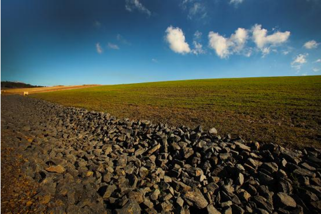
Plate 5 - Progressive rehabilitation landform – with topsoil and grassed and preliminary shaping.
