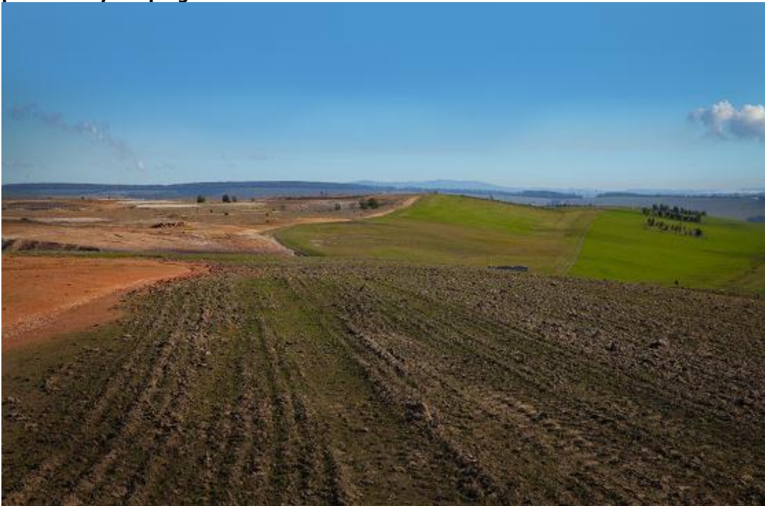
Plate 5 - Progressive rehabilitation landform – with topsoil and grassed and preliminary shaping.
