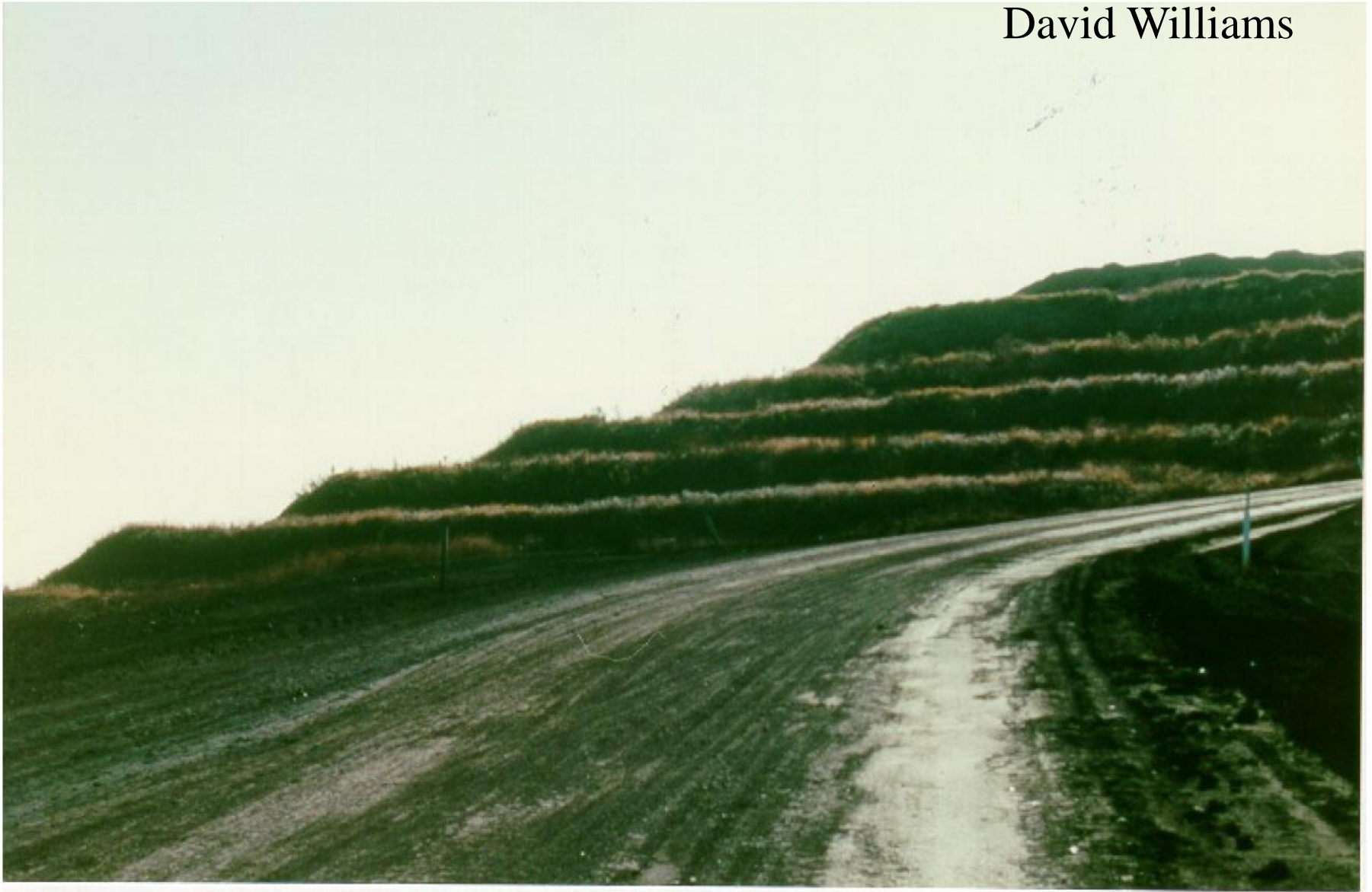
Figure 11 Stepped coal mine waste dump slopes in Witbank Coalfields, South Africa
