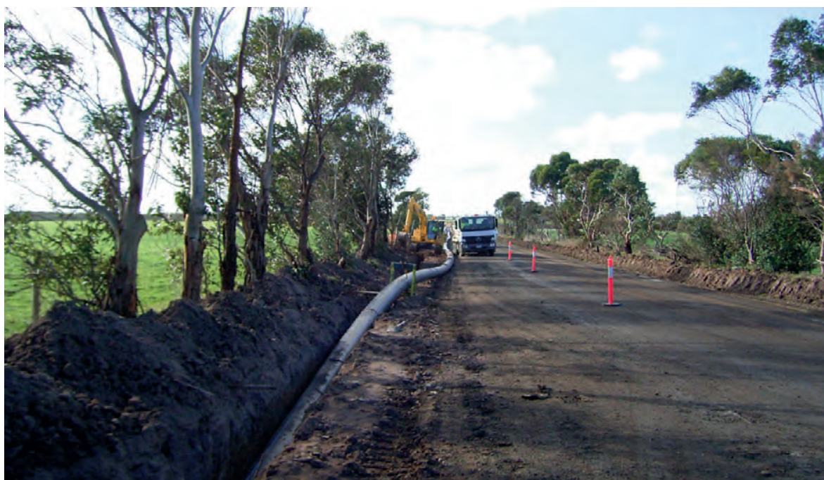
Pipe laying project, SGW
