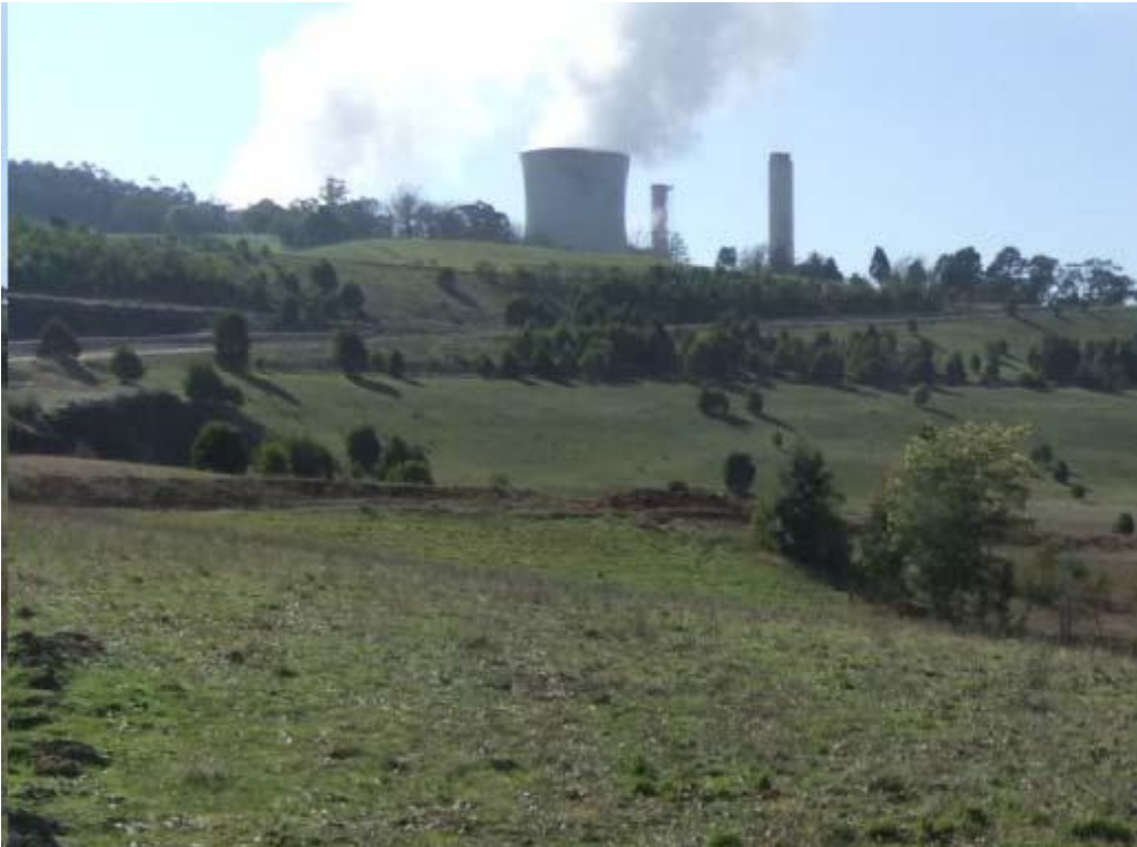
(b) Coal coverage and some woodland development taken from the Yallourn Township Field Northern Batters
