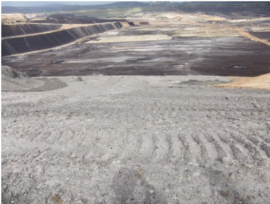
Figure 2: Topsoil Placement (Feb 2015)
