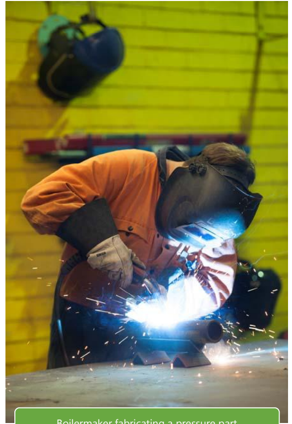
Boilermaker fabricating a pressure part
