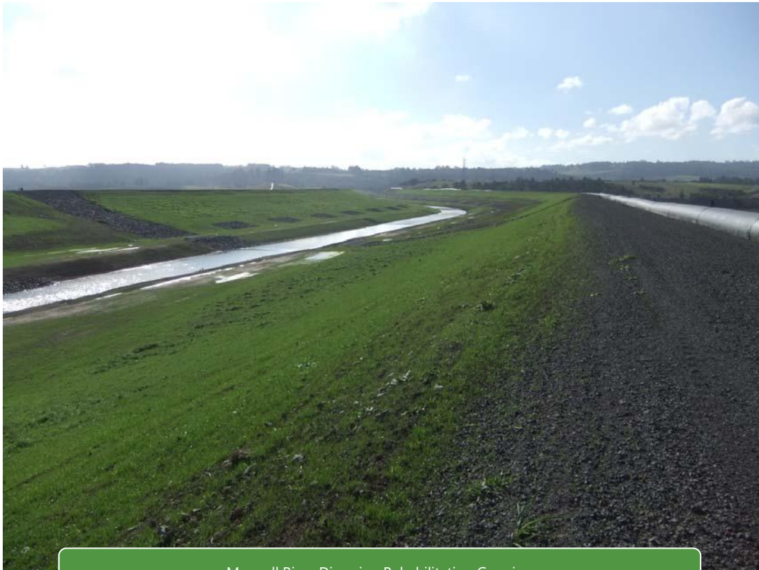
Morwell River Diversion Rehabilitation Grassing
