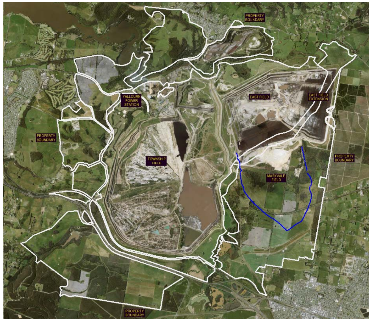
Figure 1: Aerial Photograph of the EnergyAustralia Yallourn Site - Property Boundary Highlighted in White
