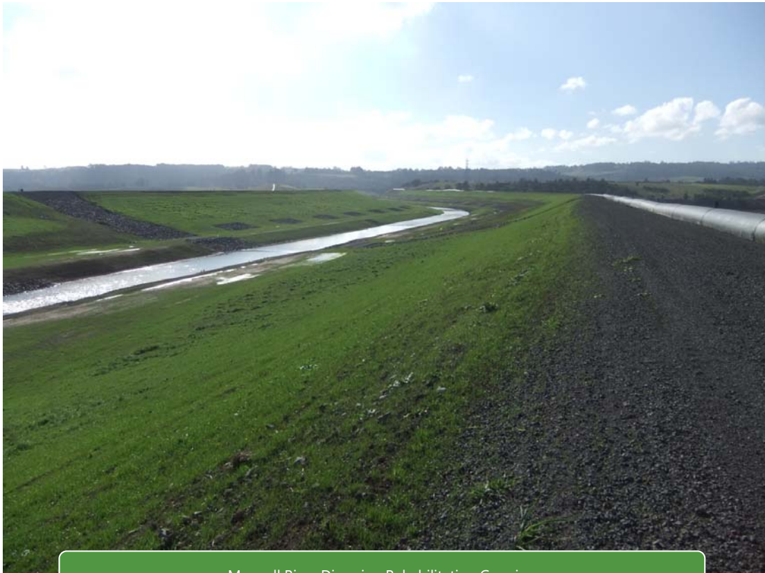
Morwell River Diversion Rehabilitation Grassing
