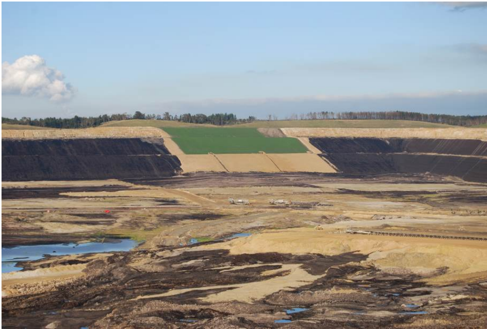
Figure 43 - Worked Out Area of the Mine - East Field Batter Rehabilitation
