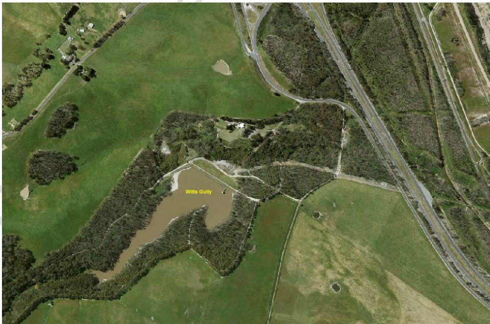
Figure 19 - Witts Gully Reservoir
