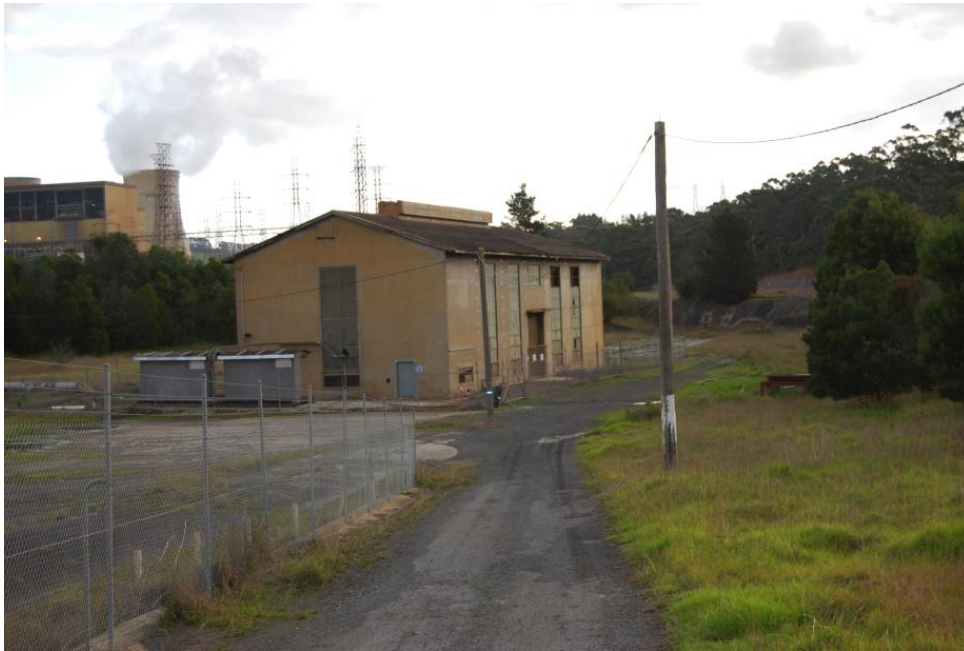
Figure 24 - Latrobe River Pump Building adjacent to the Latrobe River
