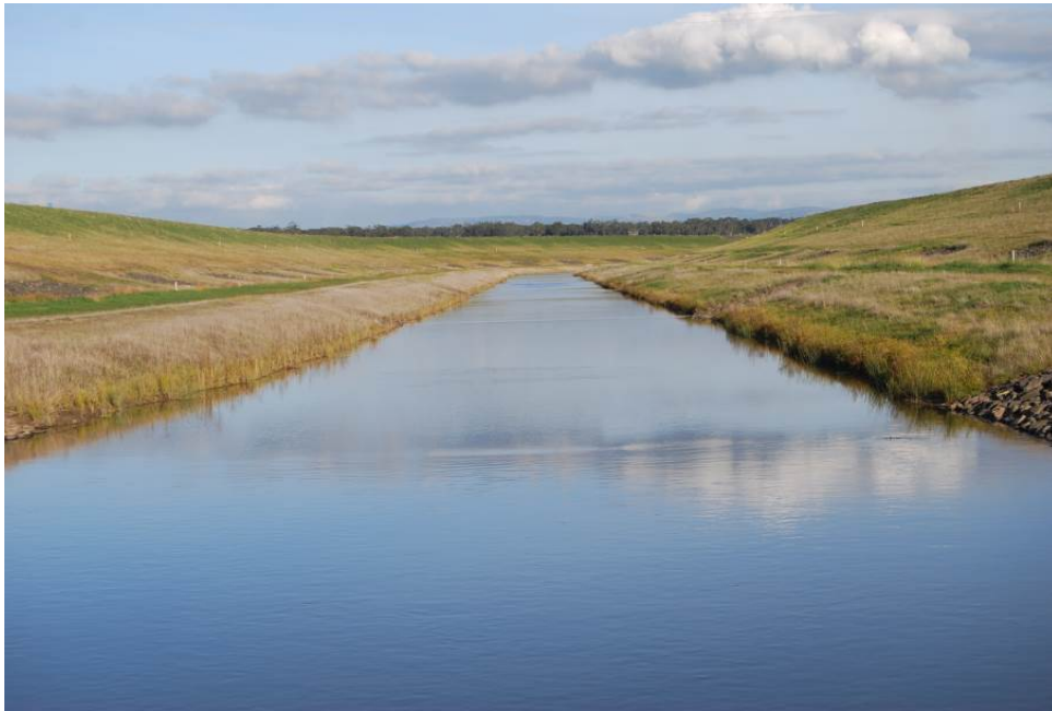
Figure 45 - Morwell River Diversion
