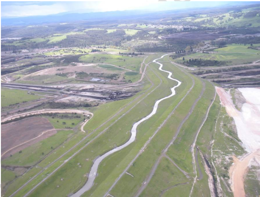
Figure 44 - Morwell River Diversion
