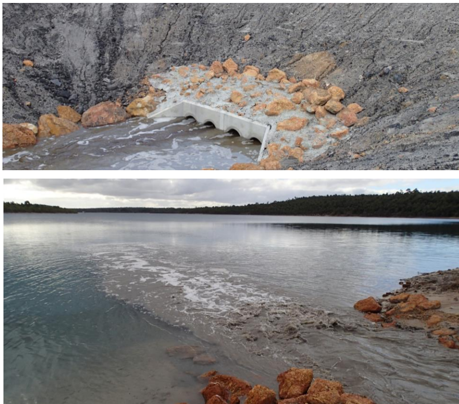
Figure 4 CRSB flow-through into Lake Kepwari in July 2013
