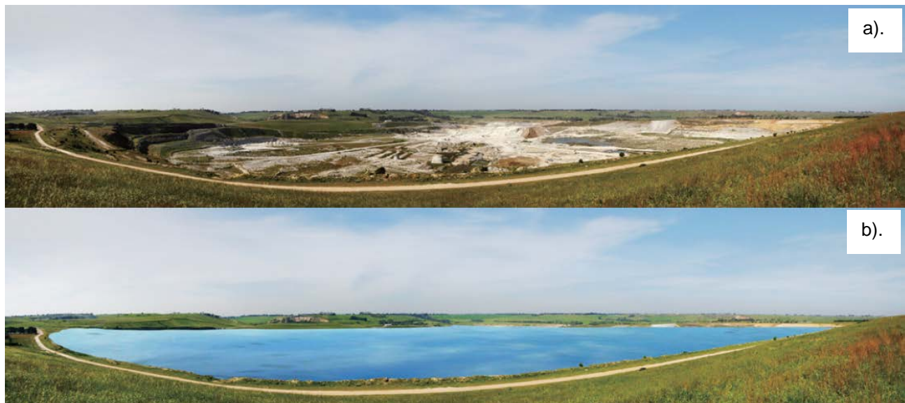
Figure 4: Artist's impression of the Batesford South Pit Lake at completion of quarrying and once groundwater equilibrium and filling is complete.
