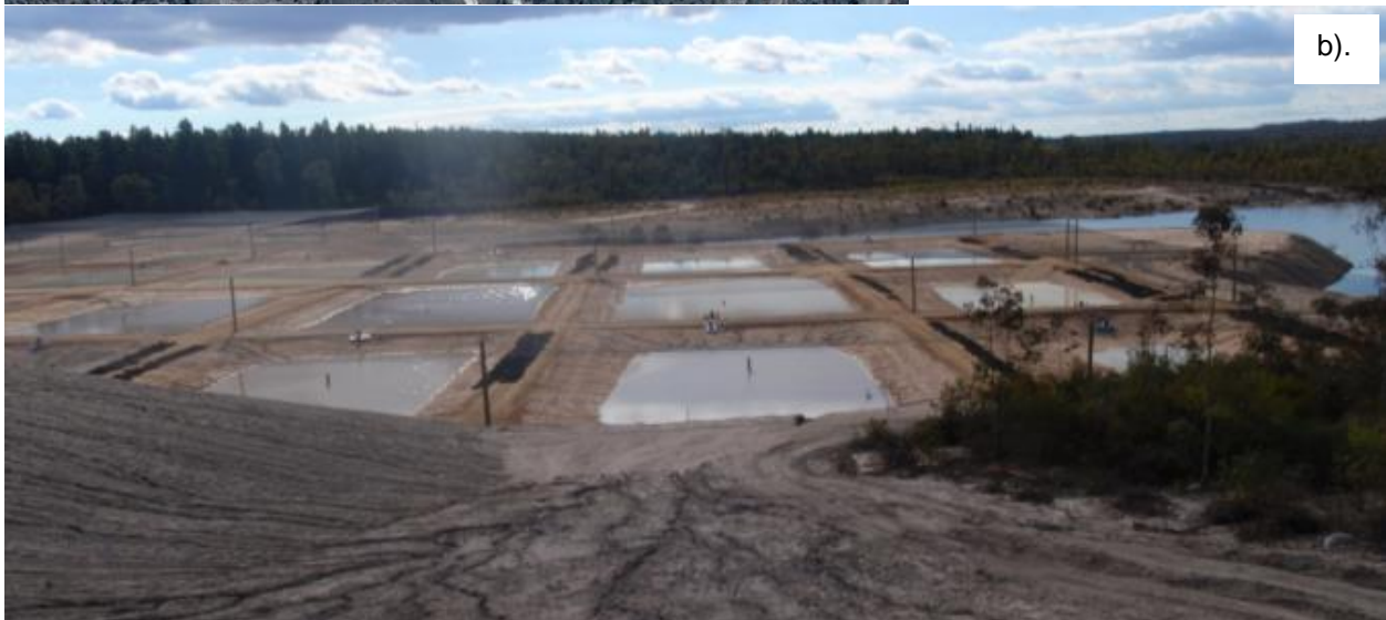
Figure 3: The Ngalang Boodja Mine Lake Aquaculture Project (a) aerial view (Nearmap) and (b) side view at Yancoal Premier Coal Ltd in Collie, Western Australia.
