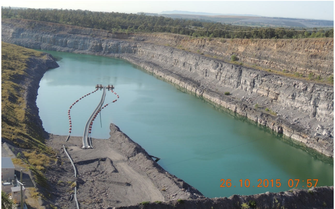
Figure 1. Glencore Ravensworth West void pit lake, Upper Hunter Valley, NSW currently being used for water transfer and storage prior to conceptual closure planning and rehabilitation works.
