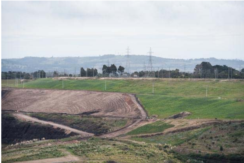
Figure 10: Northern Batters rehabilitation works in progress – late 2014/2015
