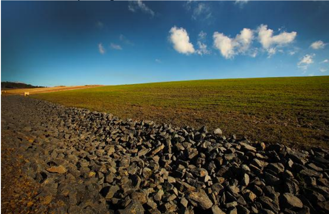
Plate 5 - Progressive rehabilitation landform – with topsoil and grassed and preliminary shaping.
