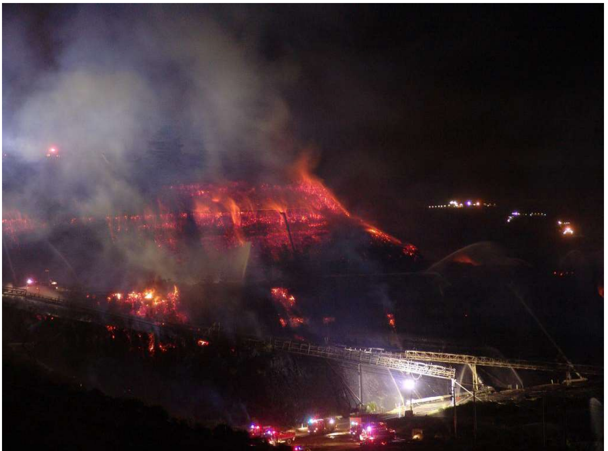
Figure 12 Recent Open Cut Fire in Coal Batters
