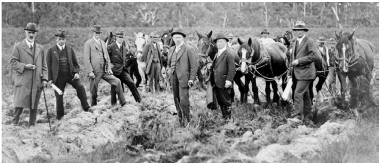
SECV Commissioners turning the first sod for the Yallourn power station, 5 February 1921
