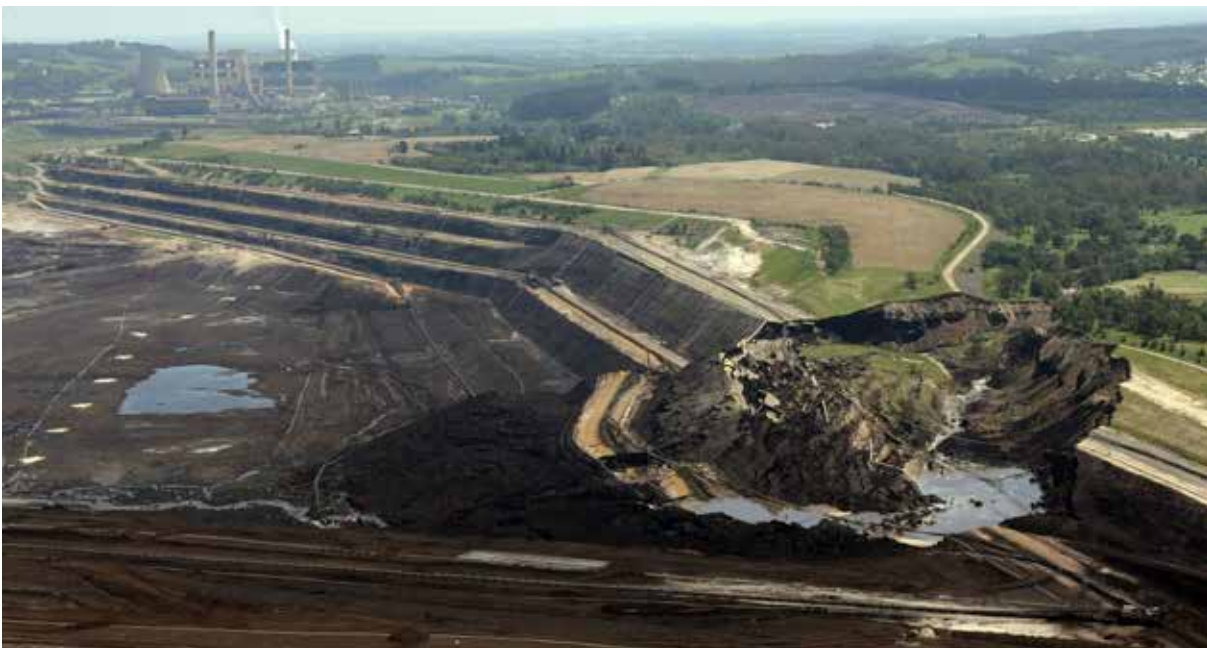
Figure 11. Yallourn northern batter collapse
