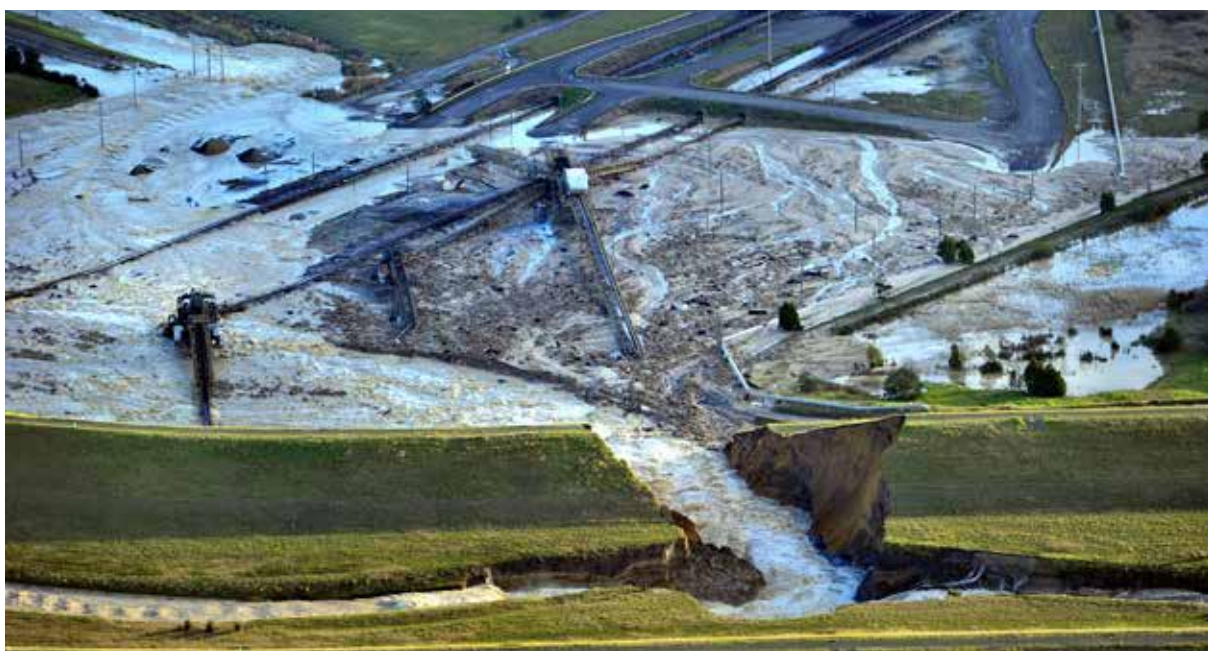
Figure 13. Morwell River Diversion failure
